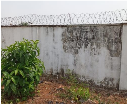
Plate 1: Wall Preparation of the college fence
