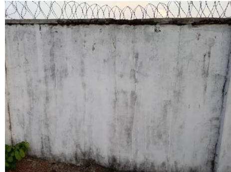
Plate 2: Priming the wall of the college fence
